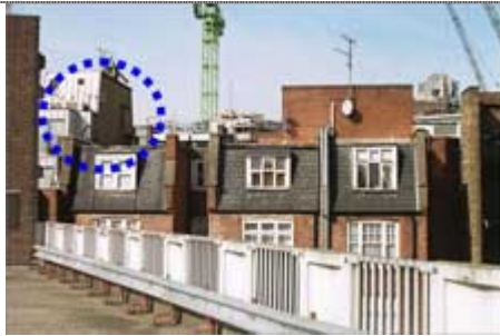
Back of Jefferson House – July 2002
